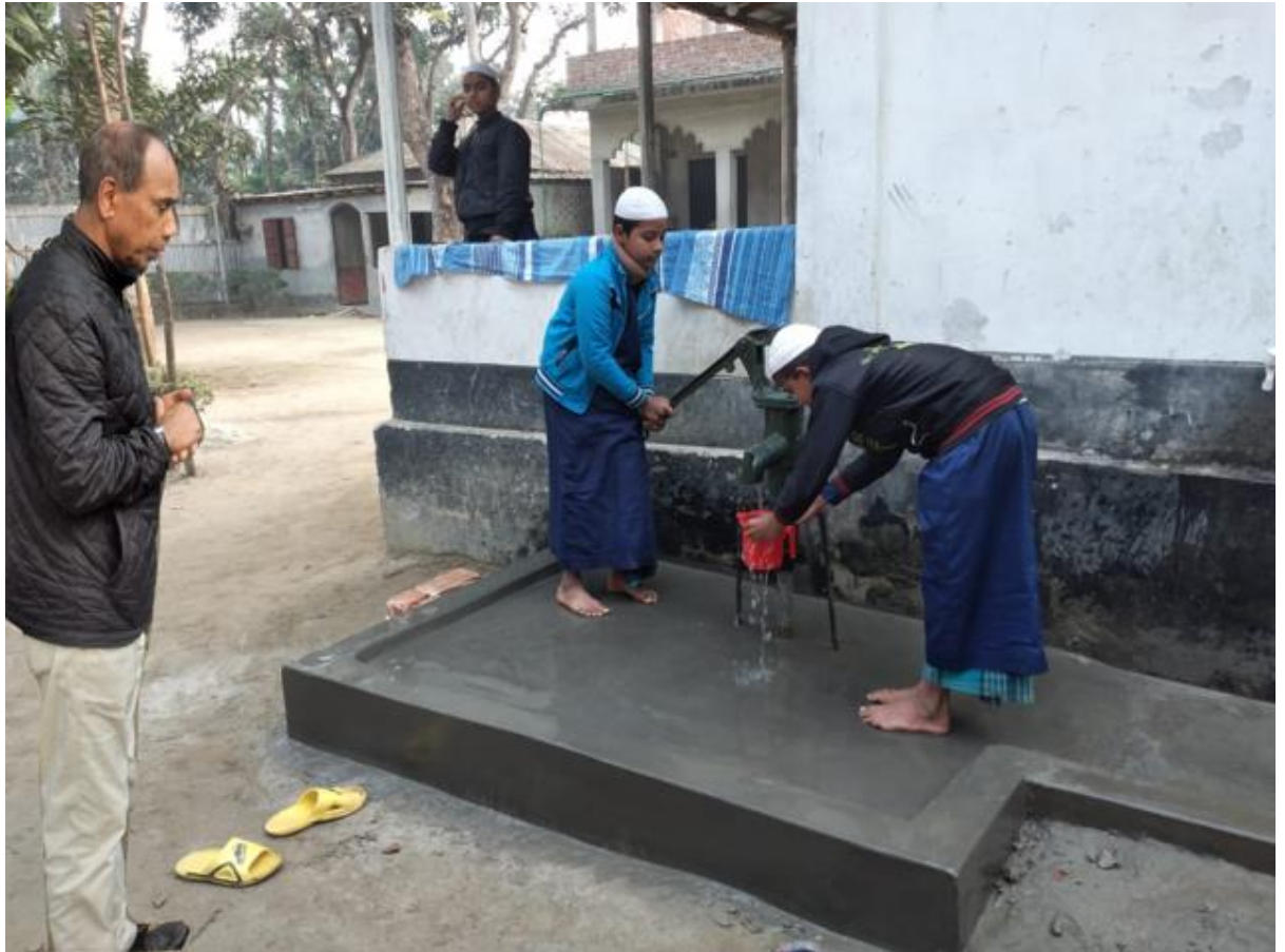
Example of a new tube well installation
